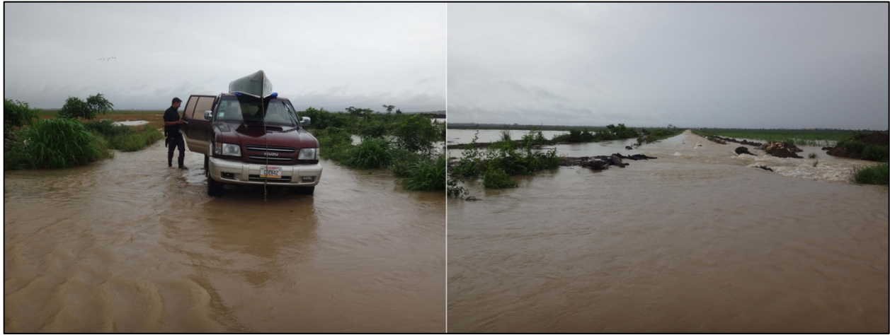
Figure 2.13 Flooding and washed out roads south of Labouring Creek (photos by J. Ramos)
