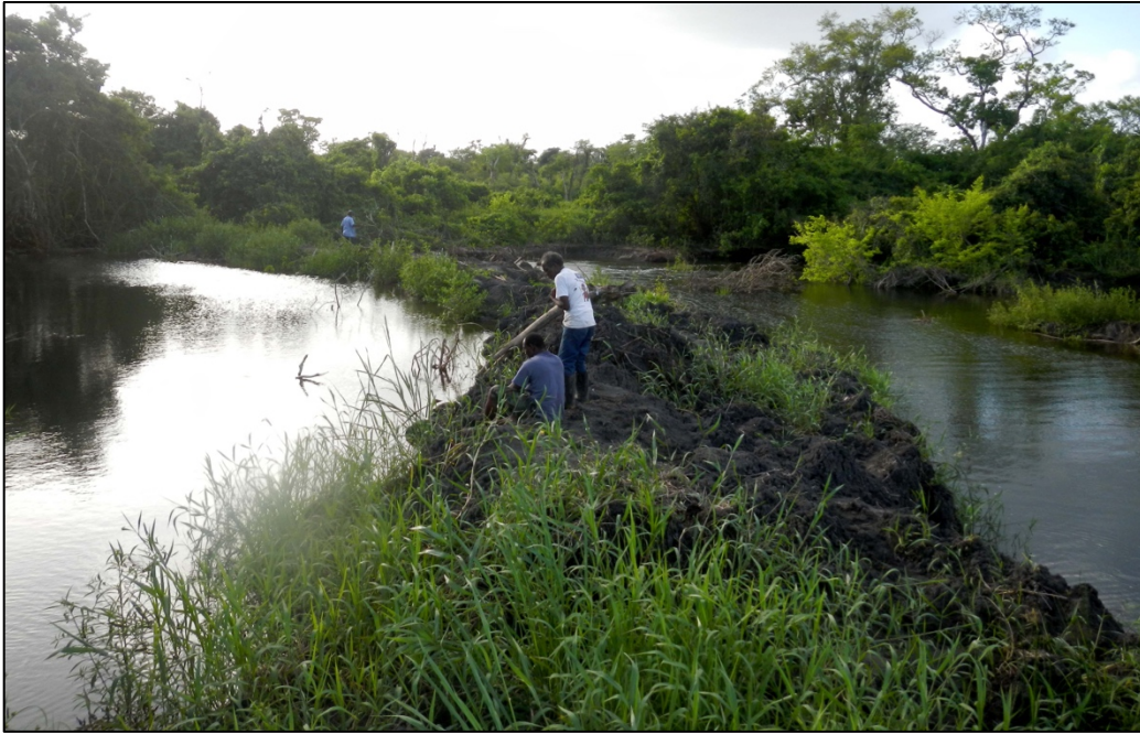
Figure 2.18 The earthen dam blocking flow from White Water Lagoon to Freshwater Creek and diverting it to irrigate sugar cane fields to the south (photo by A. Gantos)
